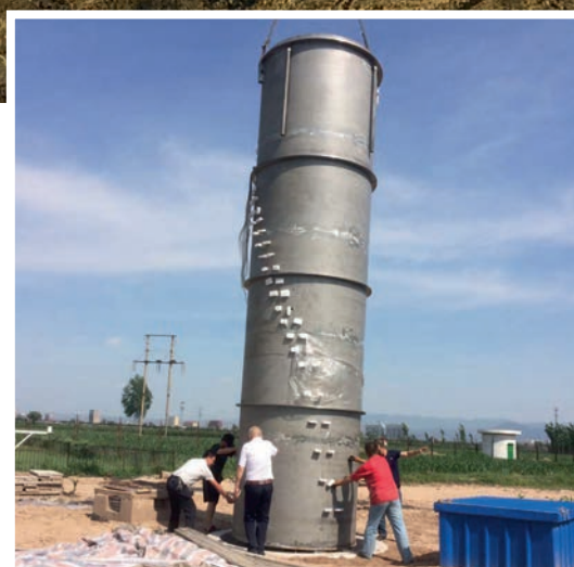
Static installation of PICO probes in an 8m deep lysimeter system in China (in operation, during installation, during the installation of the towers)
