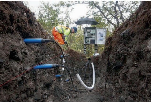
Installation example close to the surface including cabling at the data station
