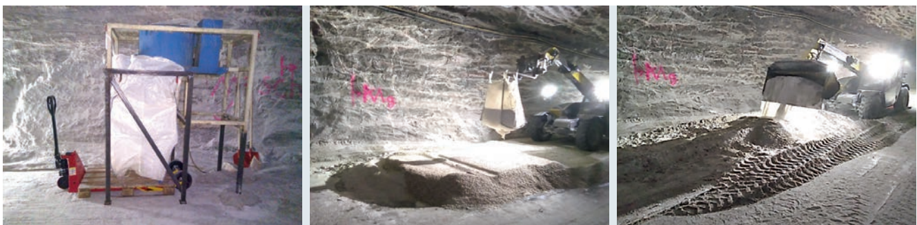
Three phases of mixing a structurally stabilized salt grit backfill
