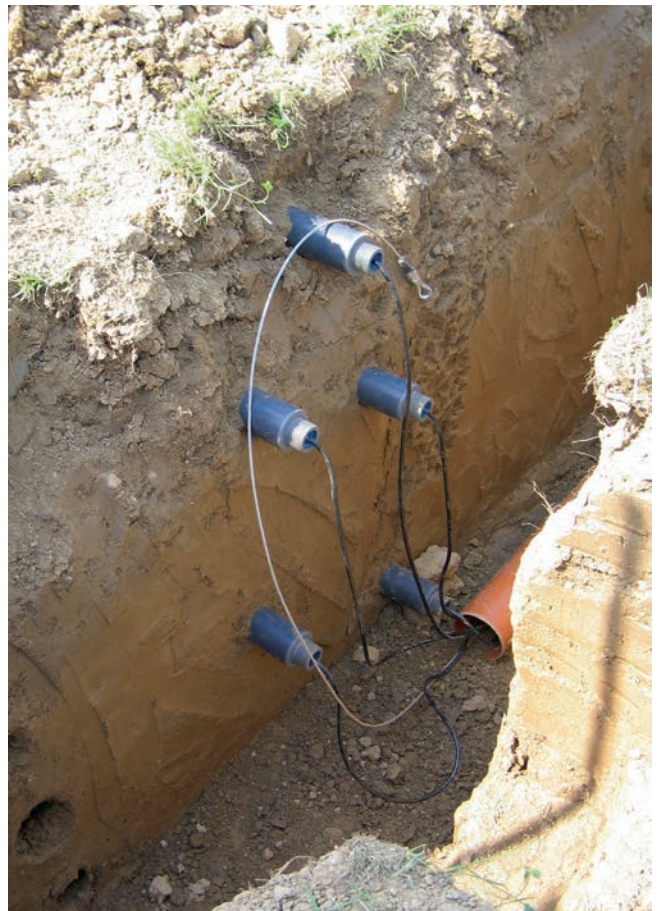
Example of the installation of PICO64 in an undisturbed subsoil
