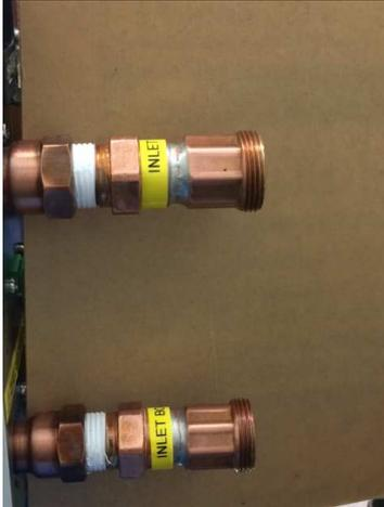
Locate the FLUID INLET distribution pipe. Install onto the interconnect pipes.
