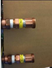
Locate the FLUID INLET distribution pipe. Install onto the interconnect pipes. Using one ranch fixed position on the interconnect pipes, and the other ranch torque carefully at the distribution pipe.
