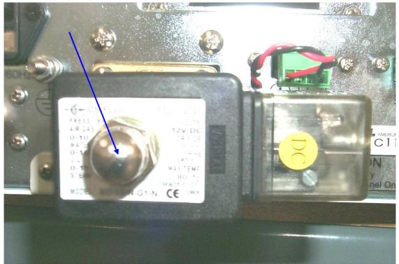
8) Now the rubber diaphragm has been replaced and the load is ready for operation.
