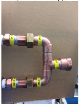
Install OUTLET TOP interconnect pipe to female threaded pipe at PLW rear panel. Install OUTLET BOTTOM interconnect pipe to female threaded pipe at PLW rear panel. Using one ranch fixed position on the female threaded pipe at PLW rear panel, and the other ranch torque carefully at the interconnect pipe, Tighten the male end connection into the mating female end connection until hand-tight approximately 2 threads. Then tighten the male end connection until wrench-tight approximately 2 threads.
