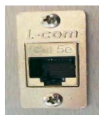
RJ-45 Network Connection
